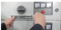
Press the unlocking button and then the rocker can be rotated clockwise
