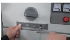
Press the unlocking button and then the rocker can be rotated anti-clockwise
