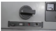
The moving button shall be turned to right
