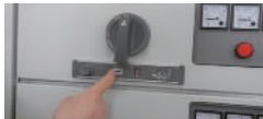
Turn the moving button left to lock the unlocking button and rocker hole
